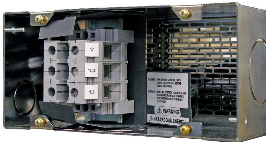
Figure 17 - Three phase, Delta AC feed connection
